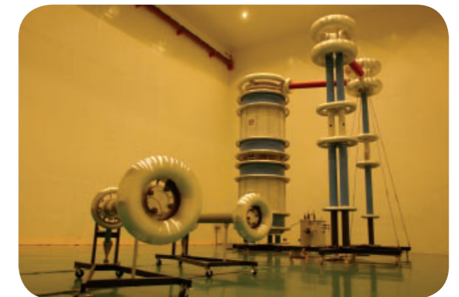
High voltage testing hall
